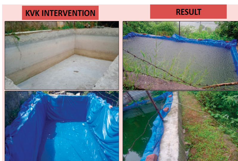
Renovation of rainwater harvesting tanks at Poonch district, Jammu & Kashmir
