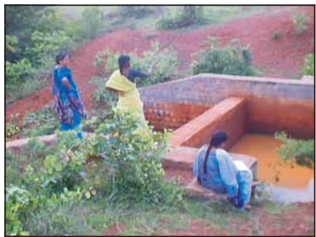
Farm woman, a beneficiary of SHG 'Sangam', explaining efficiency of check-dam constructed by DDS at Metlakunta village, near Zahirabad
