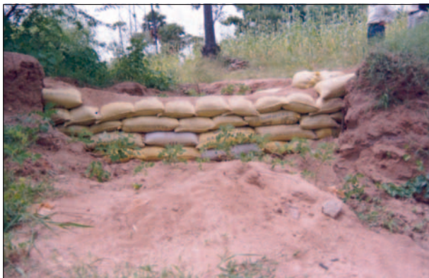
Sand bag structure as gully check
