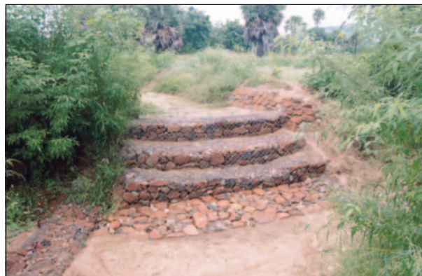
Gabion drop structure
