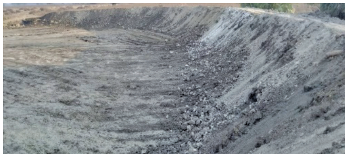
Rejuvenation of water harvesting earthen dams by desilting
