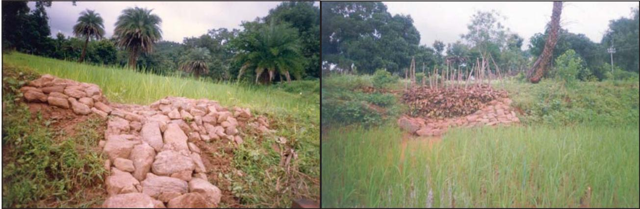
Loose boulders (left) and brush wood (right) structures across the field bund for control of soil loss and safe disposal of excess water in Sudreju watershed of Phulbani district of Orissa
