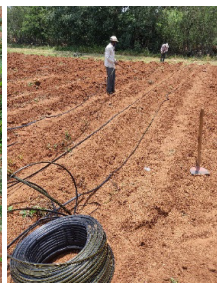
Fig. 2.2.4.2. Installing subsurface drip irrigation system
