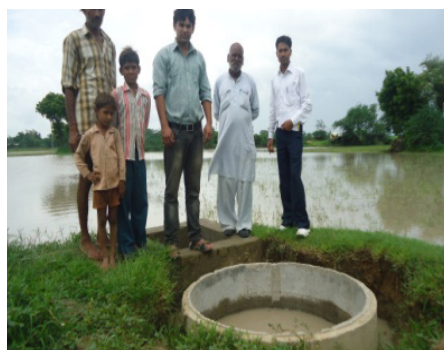
Tube well recharge structure and supplemental irrigation for wheat and mustard crops in Sitara village, Bharatpur, Rajasthan
