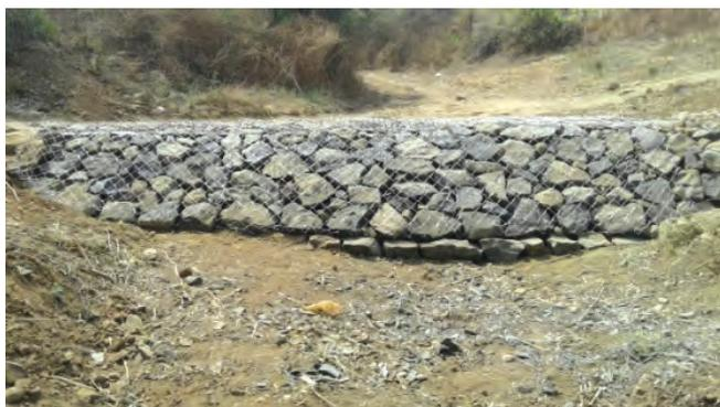
*HDPE film embeded Gabion checkdams*
