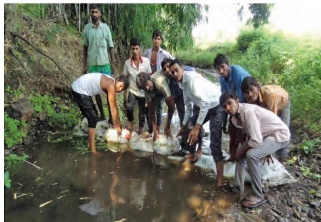
*Renovated water harvesting structure with water, polybag check dam and soybean crop in Jhabua, M.P*
