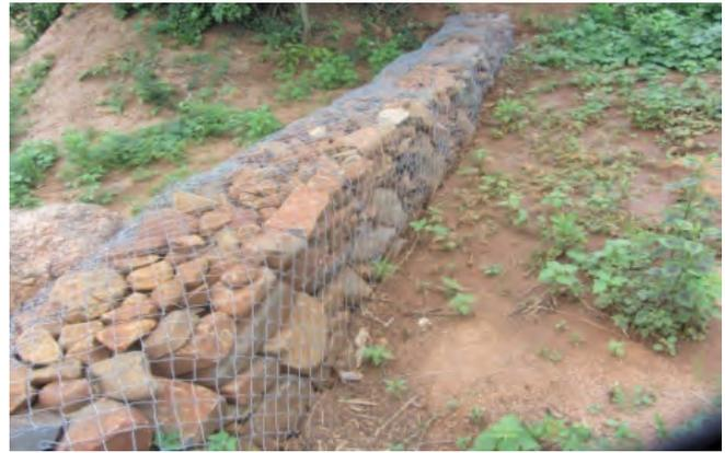
*Gabion structure for groundwater recharge*
