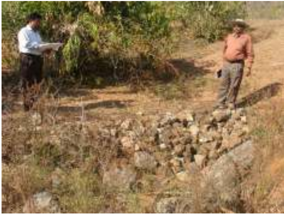
Stone gully plug for gully reclamation
