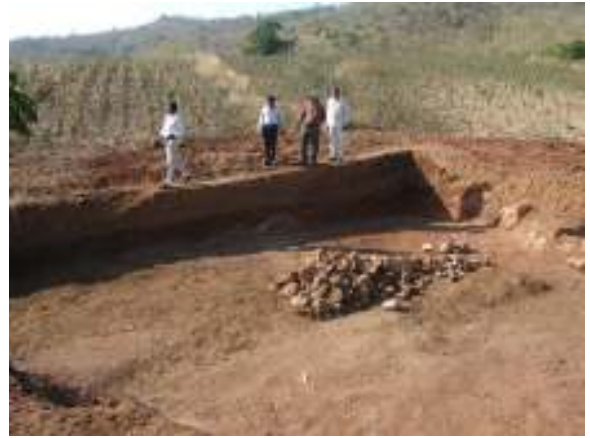
Farm pond for groundwater recharge
