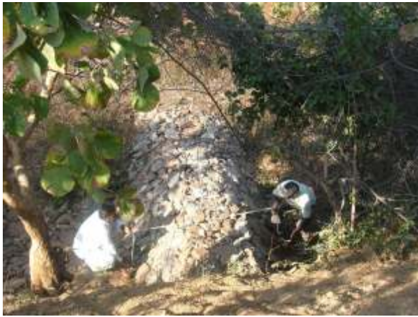
SGP across the gully
