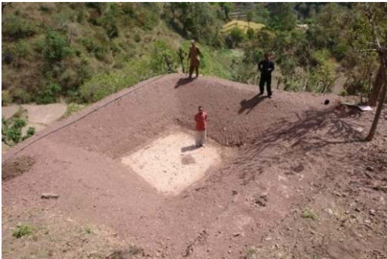
Construction of LDPE-Lined water harvesting tanks
